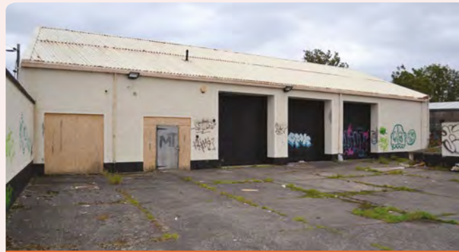
Exterior prior to renovation
