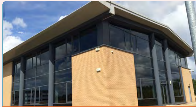
Setting provided from ground floor of office block
