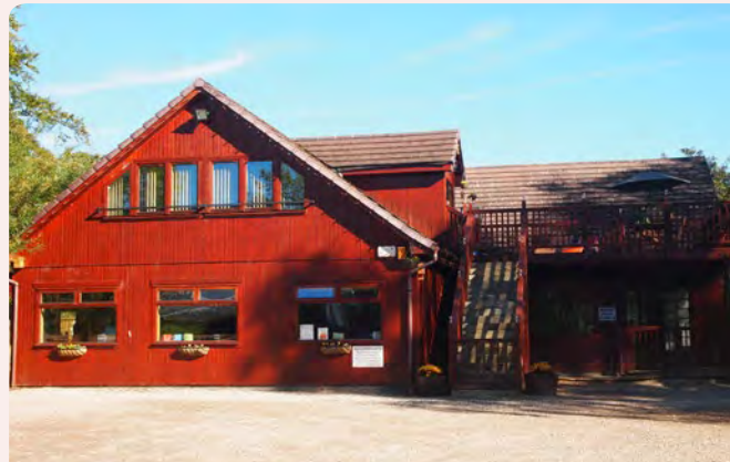
Setting provided from the ground floor of building which was previously a coffee shop
