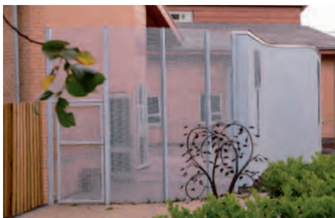
Fine mesh fence at St. Catherine's, Doncaster.
